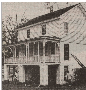
Tavern Museum Before Renovation
