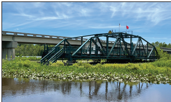
Unique swing span 1936 Walkerton Bridge preserved when current bridge was built
